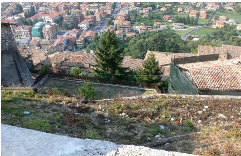
Figure 6. Situation of the terraces before the intervention
