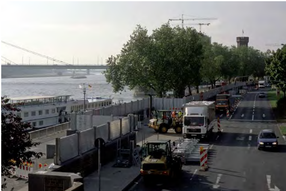
Image 9. Mobile wall spill barriers can be used to accommodate the complex environmental feedback loops operative at both normal water levels and during flooding. Köln, Germany
