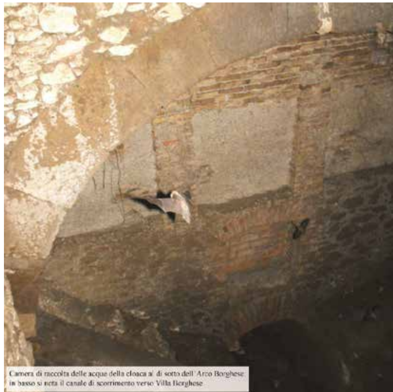
Figure 7. The sewage collection room under the Borghese Arch. Water flows toward Villa Borghese in the culvert visible at the bottom (Photograph by the Author, 2017).
